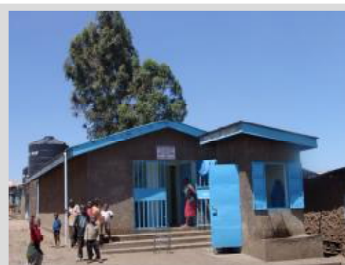
Communal toilet/washing block in Kenya:
