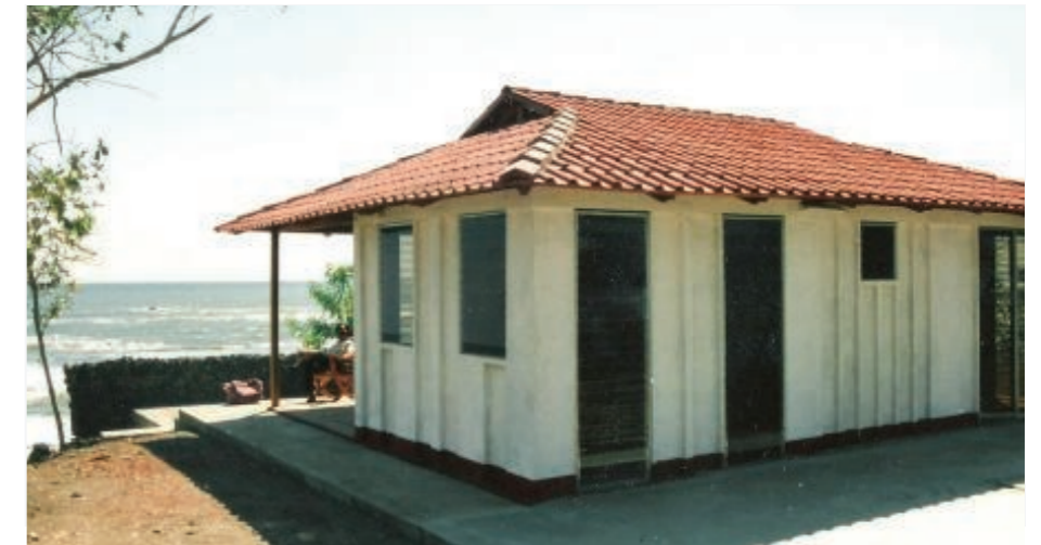
Micro-concrete roof tiles in Nicaragua. © EcoSur
