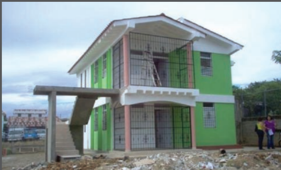
Apartment house under construction using ferro-cement in Dominican Republic © EcoSur
