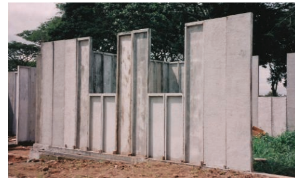
A house being constructed using ferro-cement panels in Nicaragua. © EcoSur
